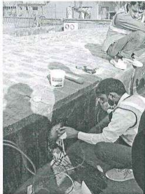
Figure 1.6 UPV Test
