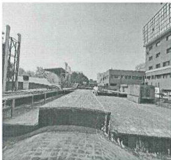
Figure 5 Brick bat Coba waterproofing over bunker roof
