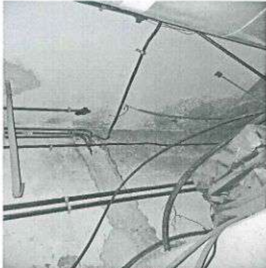
Figure 3 Dampness in Maze slab
