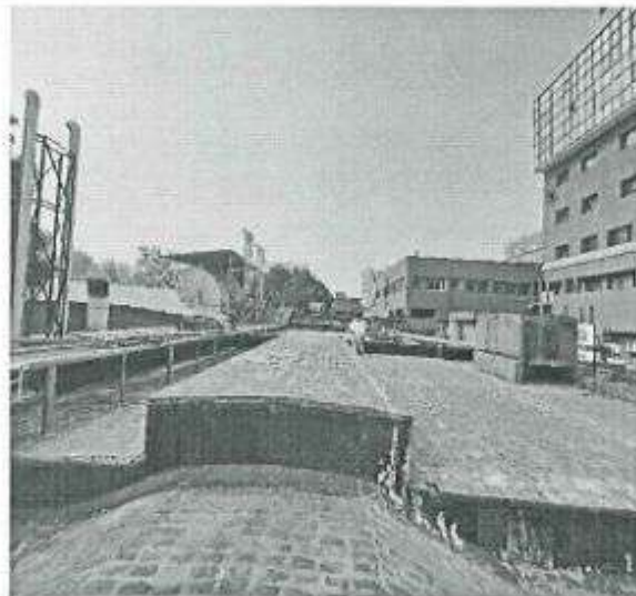
Figure 5 Brick bat Coba waterproofing over bunker roof
