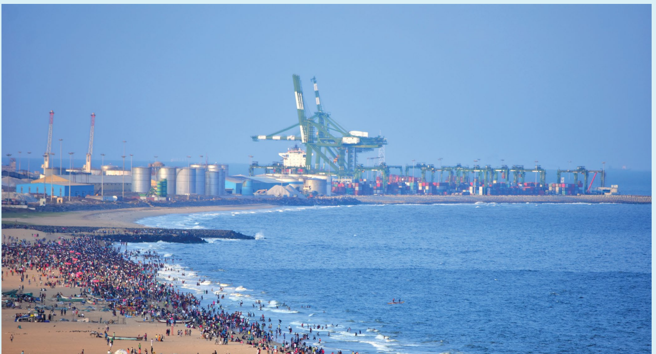
----- Image: Aerial View of Chennai Port -----
